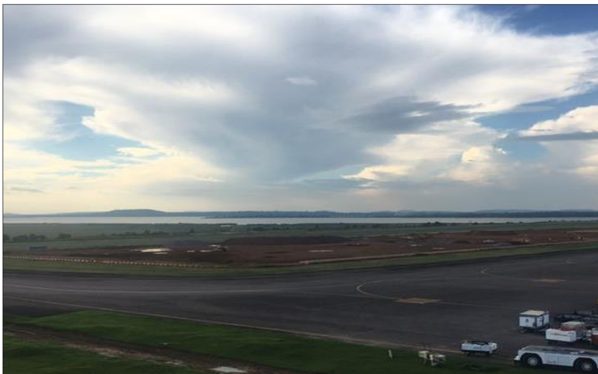
Figure 17: Apron 1 – Expansion Works (February 2018)
