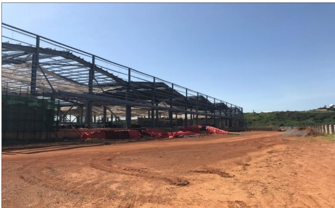
Figure 16: New Cargo Facility Construction (March 2019)
