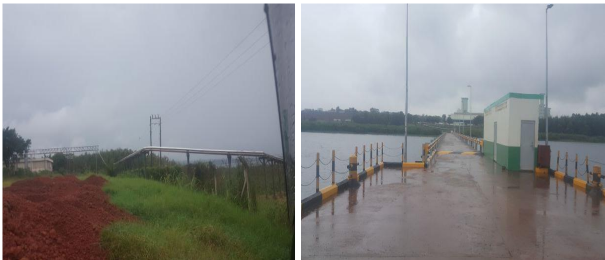
Figure 20: Bidco Palm Oil jetty
