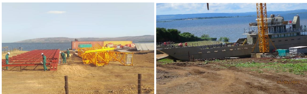
Figure 19: Veron Shipyard during construction of the 350 ton UNRA ferry
