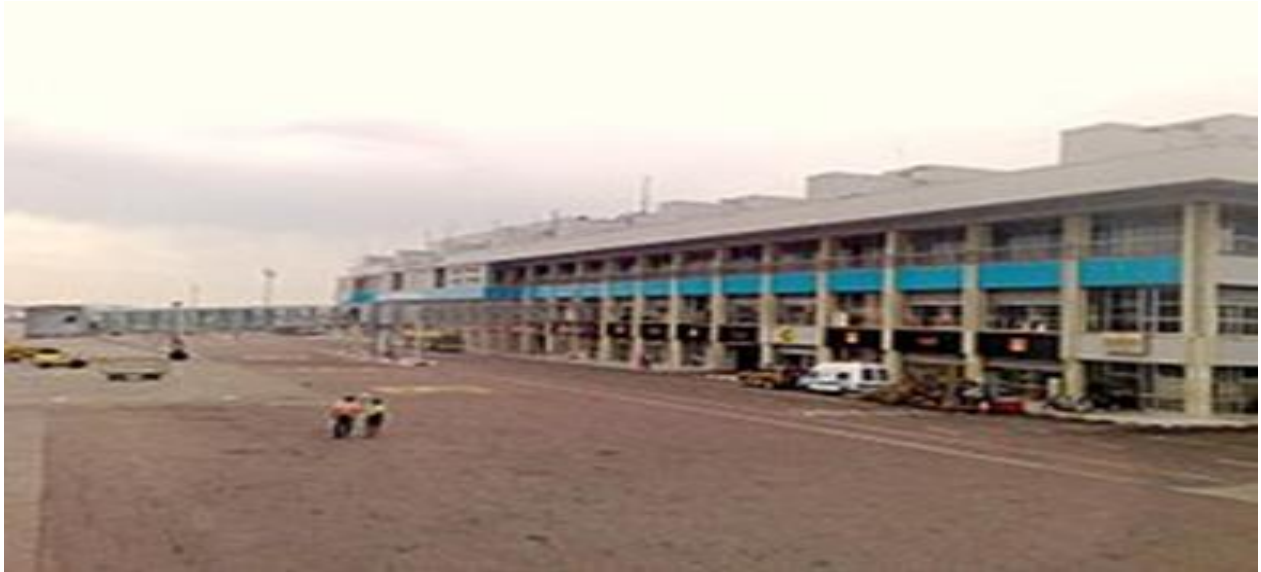
Figure 12: Entebbe International Airport
